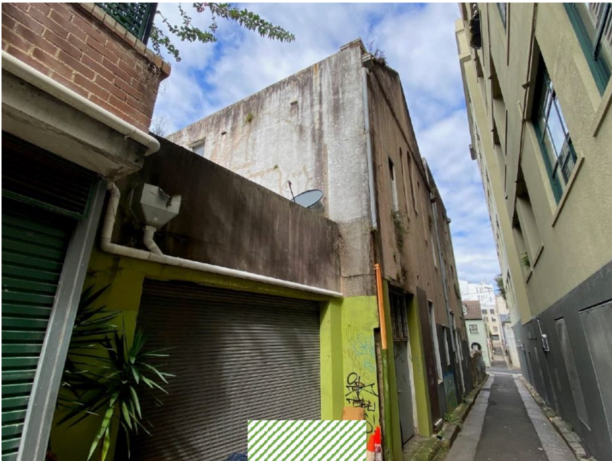
site viewed from Beauchamp Lane looking south-east
