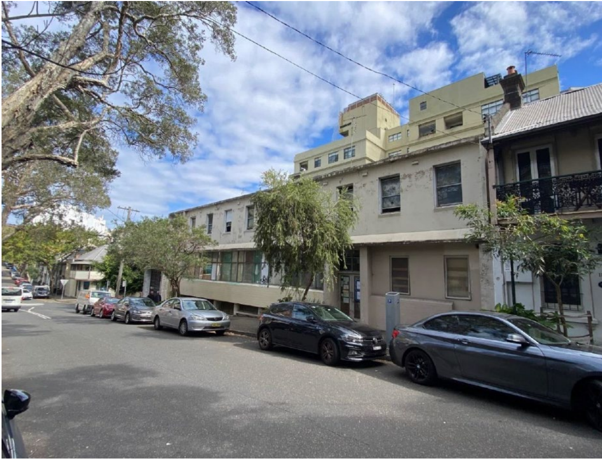
site viewed from Commonwealth Street looking south-west
