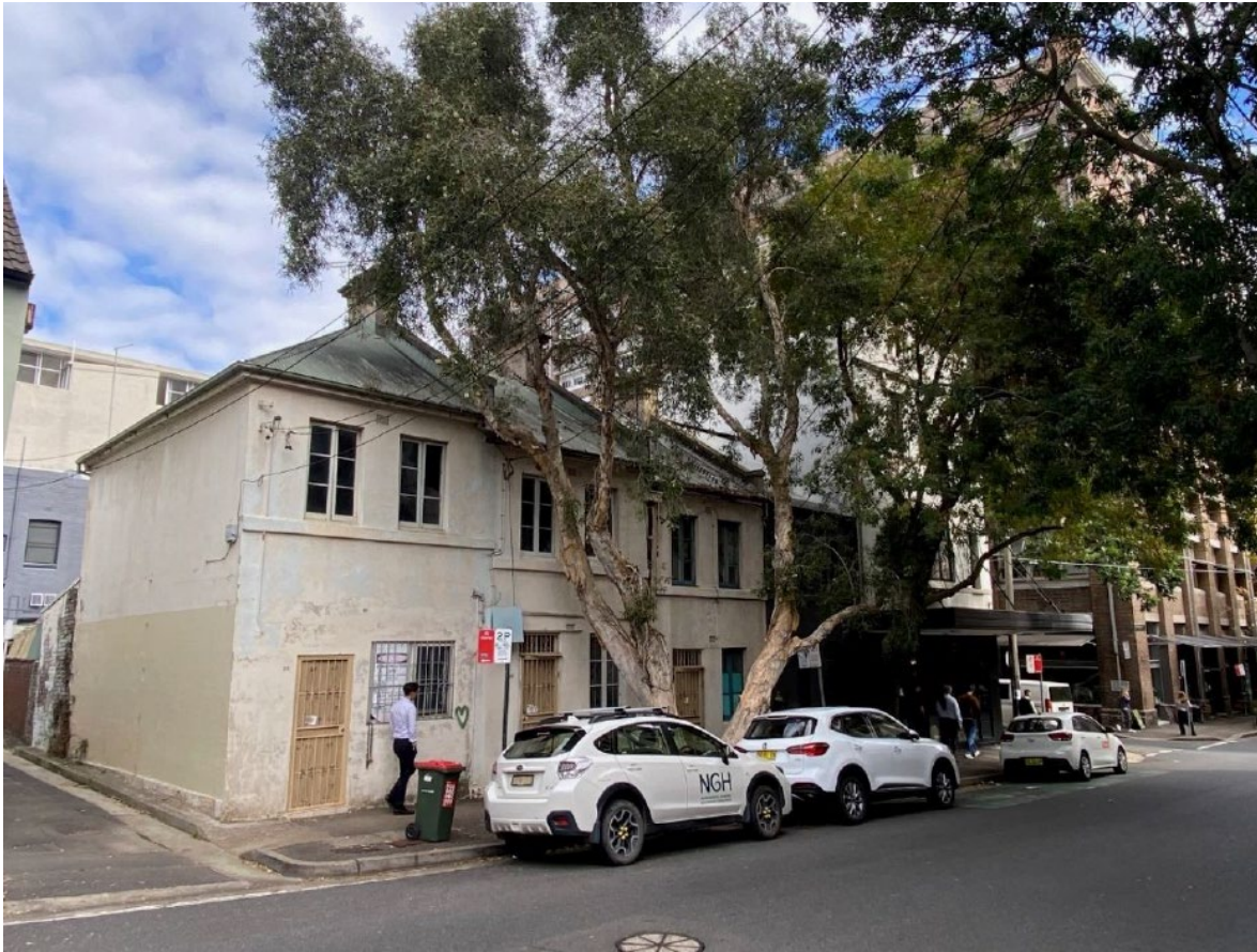
existing development on Reservoir Street diagonally opposite to the south-west
